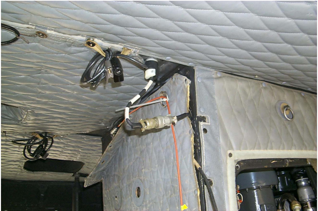
Figure 2. DC Power Cable Installation
